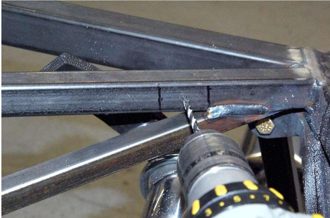
Drill the 1" tube in the middle of the tube in the middle between the rubber side marks made with a  $\frac{3}{16}$ " drill bit.
