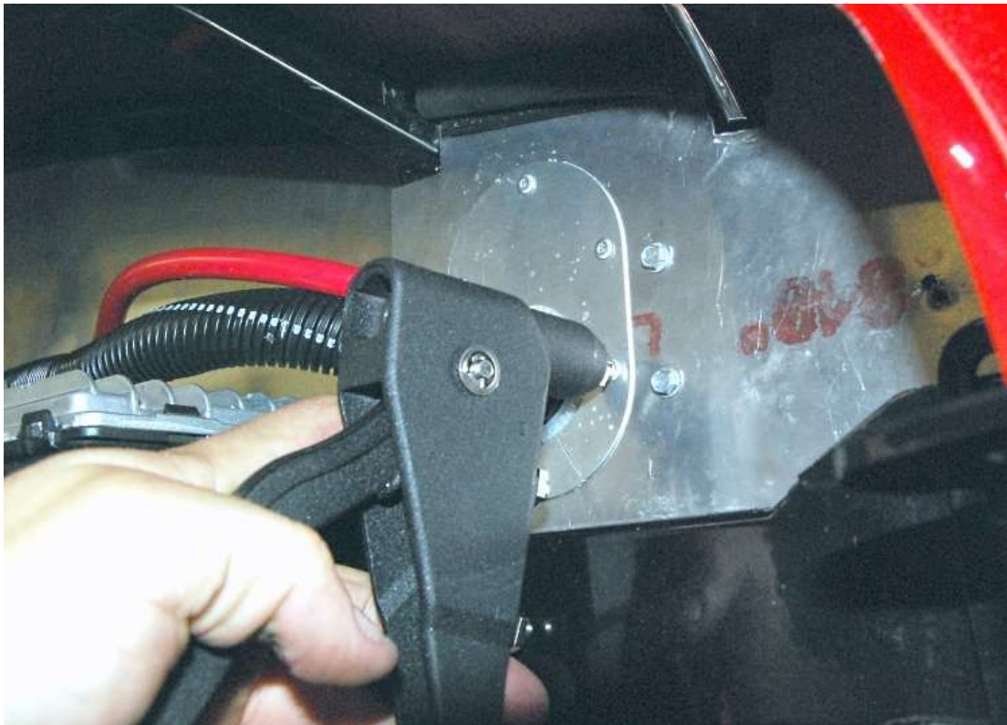
Silicone and rivet the block-off cover to the firewall extension.
