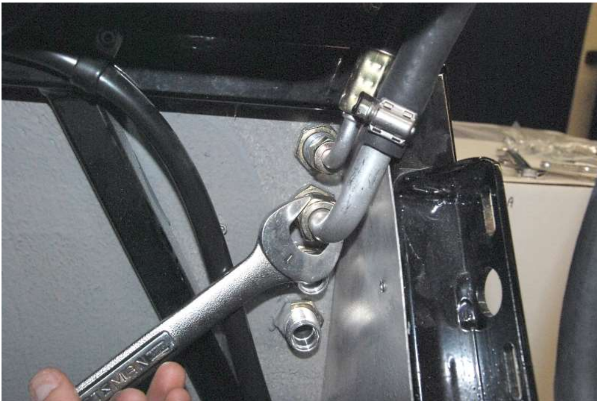
Screw on the second down inside heater fitting by hand then tighten using a 1" wrench.
