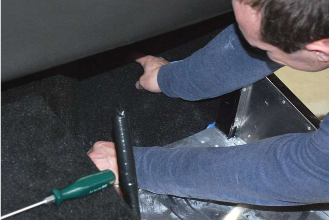
Fit and glue the lower floor sections.
