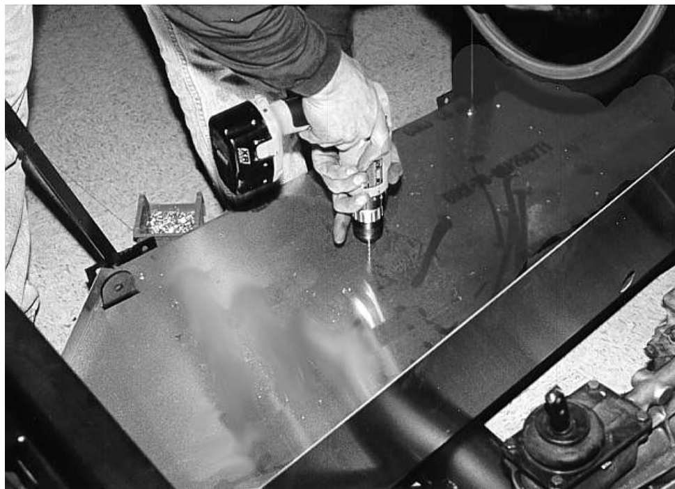
With the panel clearly marked, drill all rivet holes in advance.
