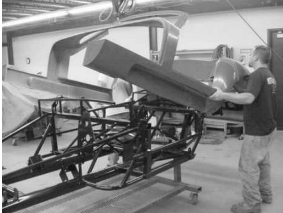
Lowering a body down onto the chassis.
