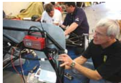
> At any one time there were three or four areas of the car being worked on, which allowed us to build it in a week. Here you can see where the MSD 6AL box and starter solenoid are mounted. The aluminum firewall should be mounted while the body is fitted to the chassis since it is a locator for a bunch of other parts. We painted the body before the build, so the firewall had already been positioned and marked.
