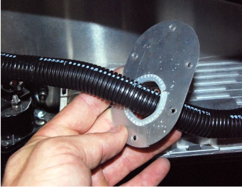
Use some grommeting from the misc. electrical components to protect the harness.
