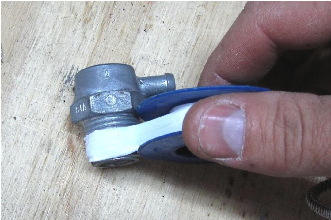
Wrap the vent with Teflon tape
