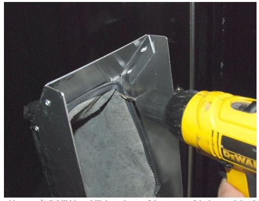
From the underside, use a  $\frac{3}{16}$  drill bit to drill through one of the corners of the boot and the aluminum.
