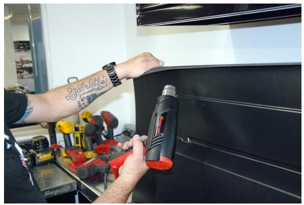
If the top flange does not sit down on the top of the door, use a heat gun or hot air dryer to bend the liner over more.
