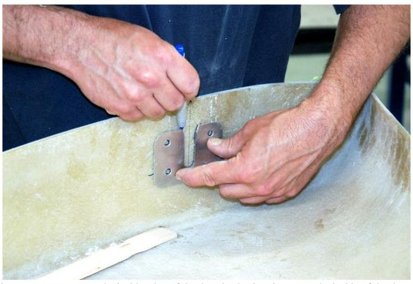
Using this measurement, trace the inside edge of the door latch trim piece onto the inside of the door skin.
