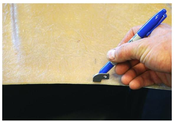
Evenly space the cowl trim mounting brackets around the hood as shown above so that the tab is flush with the back edge of the hood and mark the hole location.
