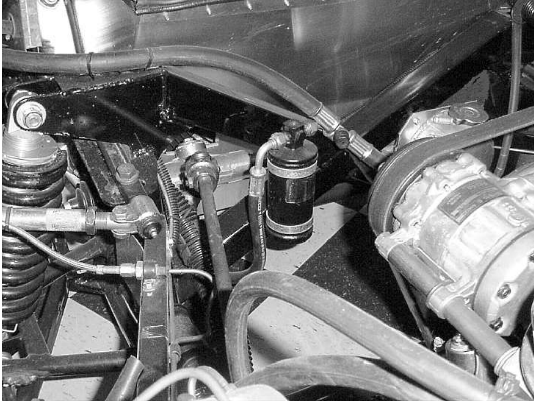
Drier mounted to the front suspension "X" with high pressure service port next to it.
