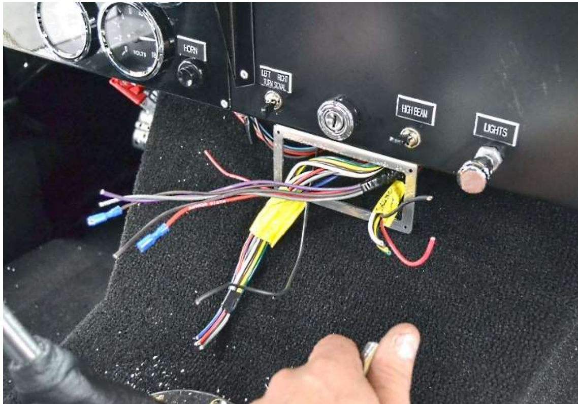
Pull the wires through the mounting bracket if used. (FFR Coupe dash shown)
