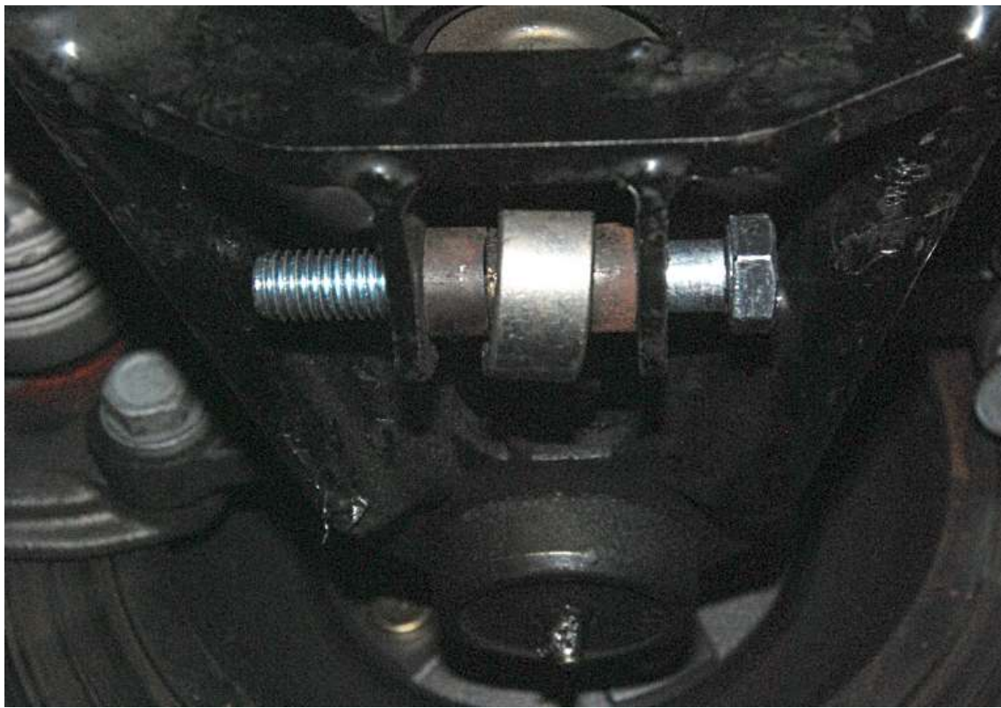
Run new \frac{1}{2} "-13 x3.25" bolts through the control arm from the front of the car back reinstalling the spacers and shock end.
