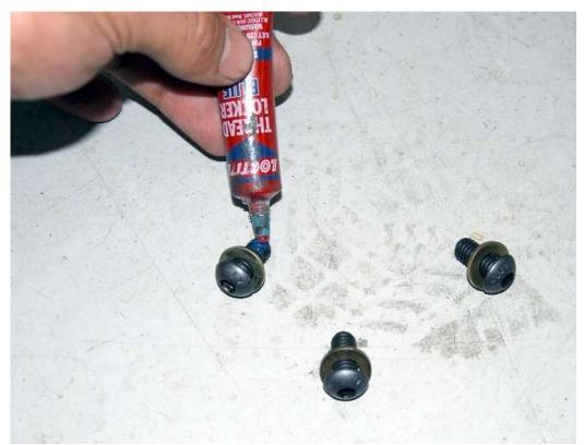
Place a washer on each of the scress then put a drop of blue Loctite on the screws.
