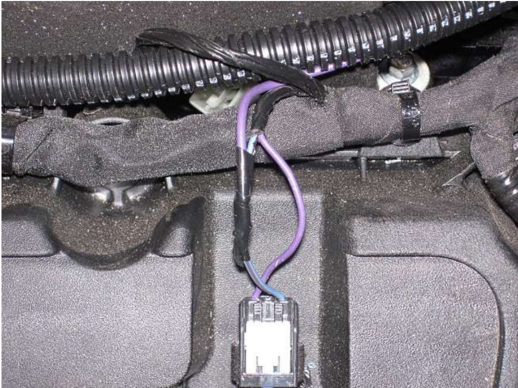
Wrap the connection in electrical tape.
