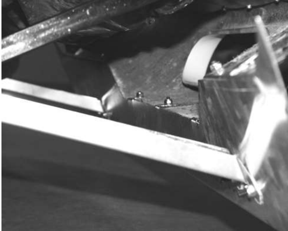
Support brace attached to Air Dam
