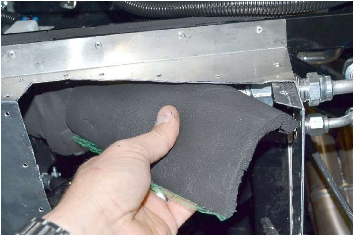
Pass the \frac{3}{4} " hose insulation over the top of the top tube in the footbox.
