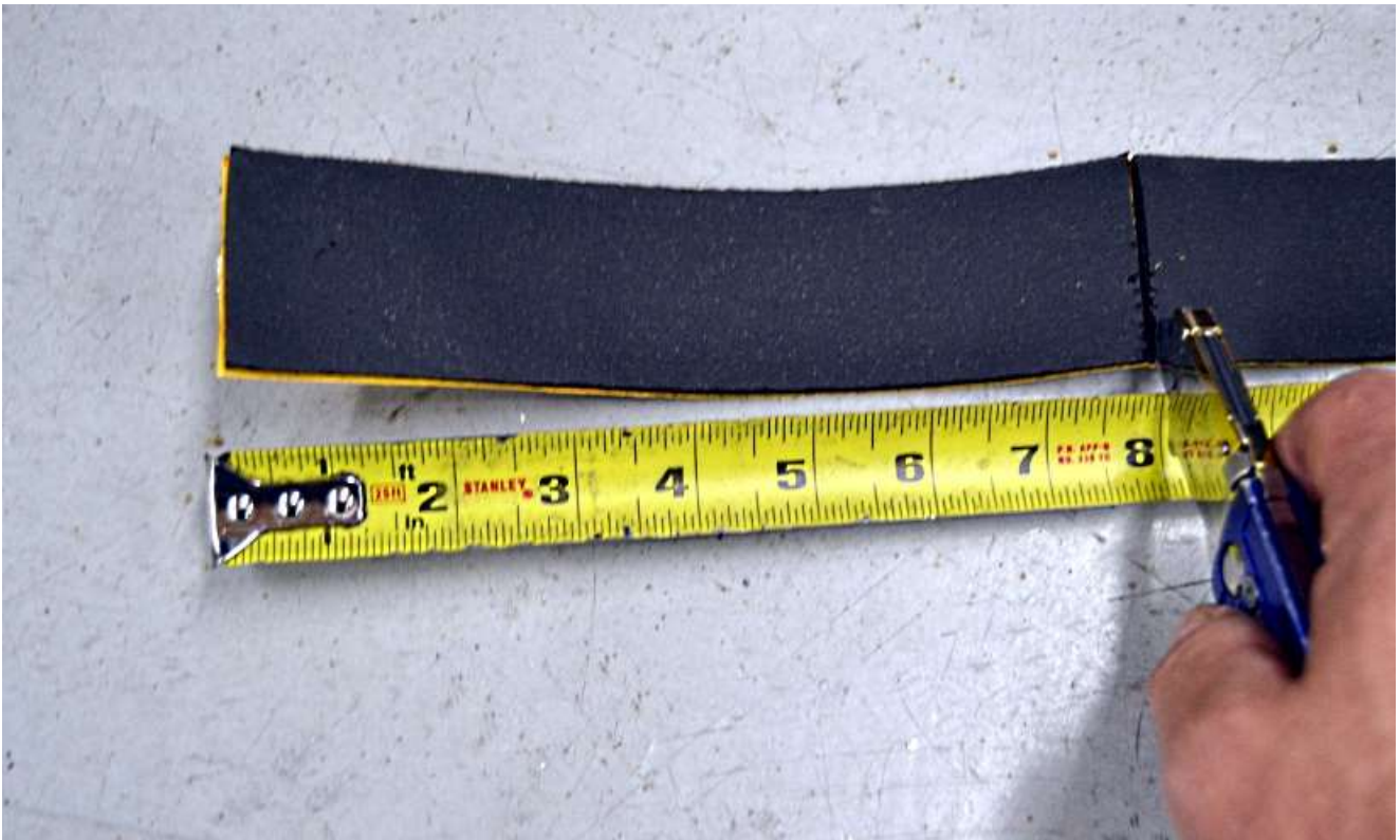
Use a razor knife to cut 8" of the \frac{1}{8} " pipe insulation.
