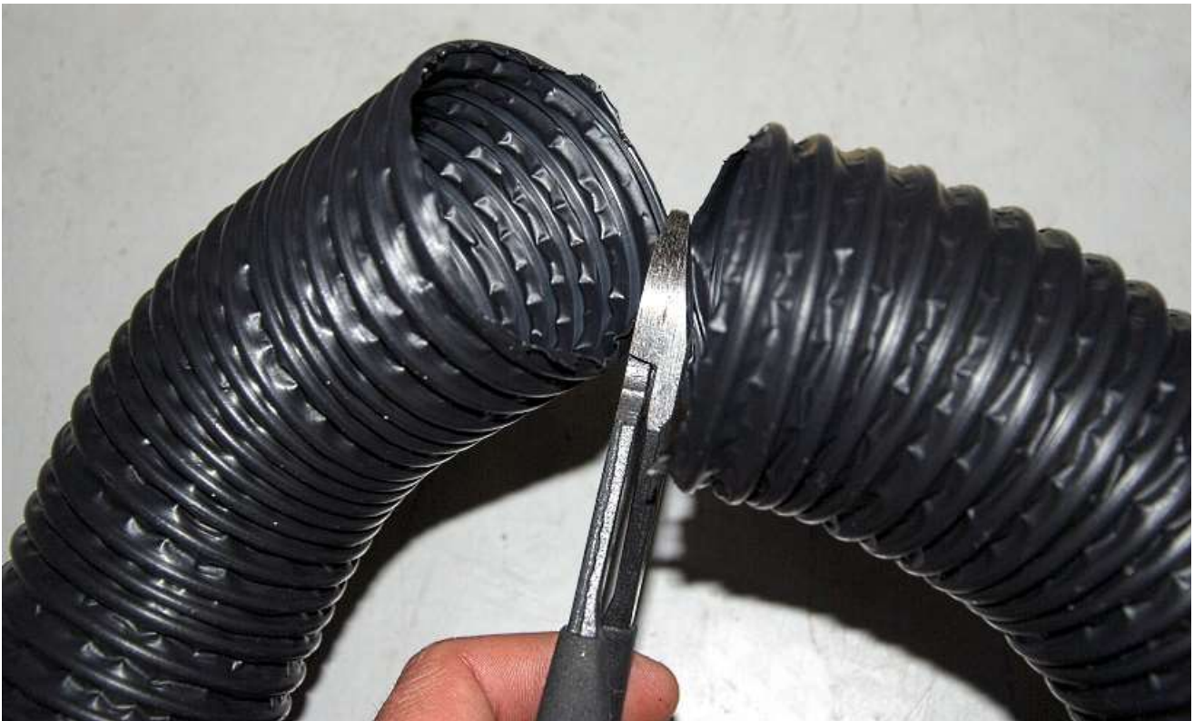
Use wire cutters to cut the hard wire.
