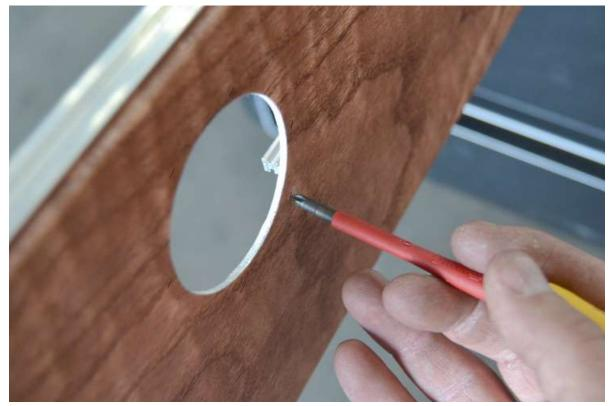
From the top side, use a Philips head screwdriver to open up the slices.
